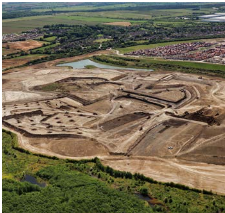
Zone 2 Earth movement works, Priors Hall – May 2020
