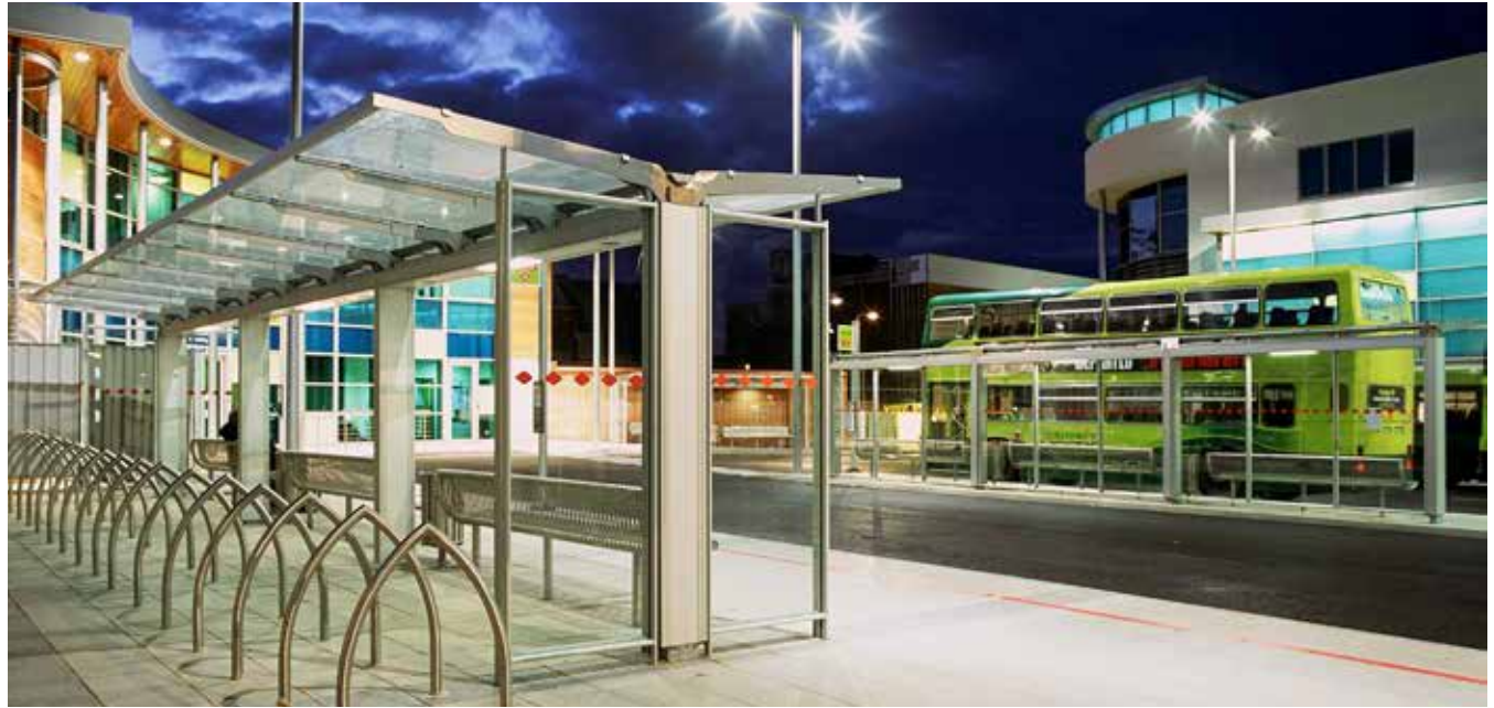
Precedent bus shelter, with seating and cycle stands (Source: Woodhouse)
