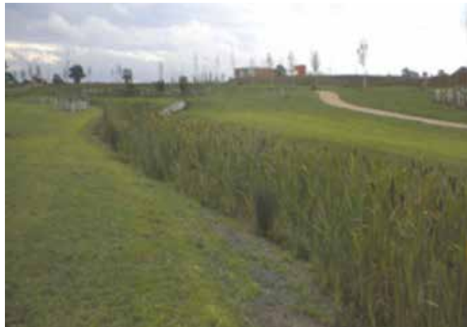
It will be possible for areas of permanent water to be kept in balancing ponds and wetlands to create habitats and encourage biodiversity while attenuating water in more extreme events.
