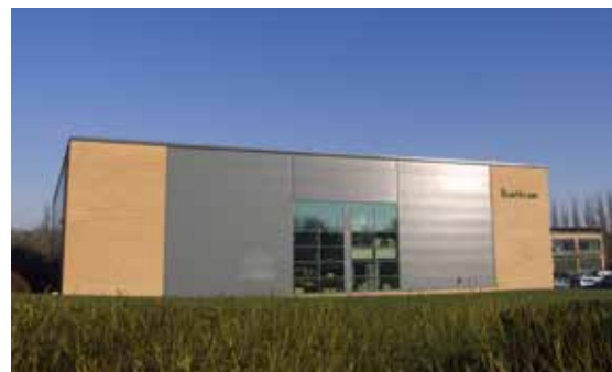
Precedent Flat Roof Industrial Unit, Knowlhill
