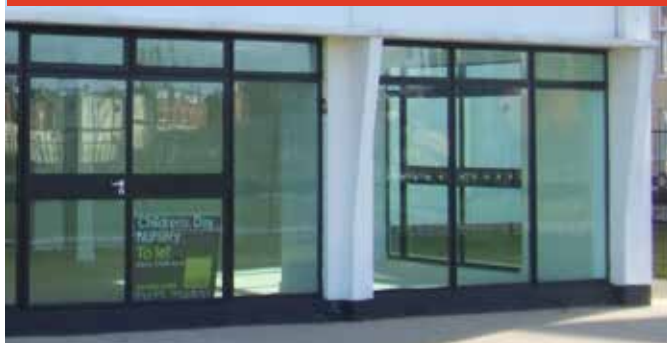
Example of a unit created to provide space for a day nursery
