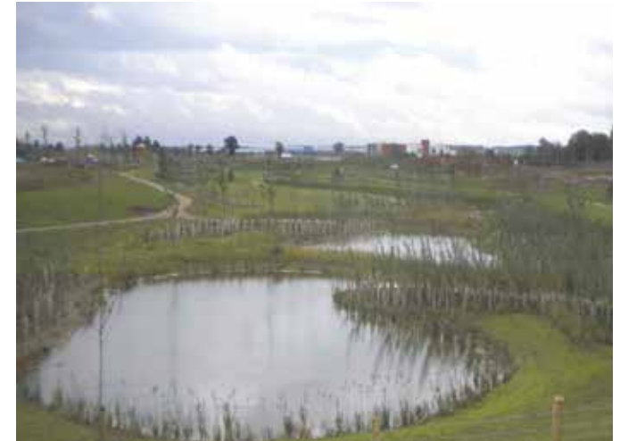
Where storage capacity is limited, the use of swales and attenuation ponds could be enhanced by the addition of a modular storage to maximise drainage/storage potential.
