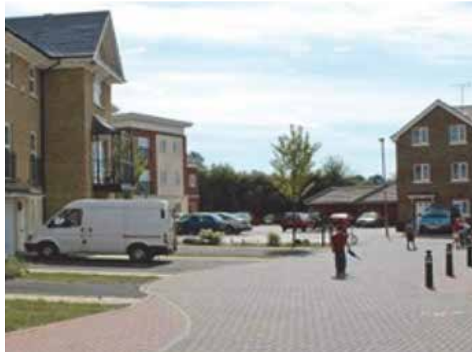
Permeable paving can be provided on parking or other paved areas within the development.
