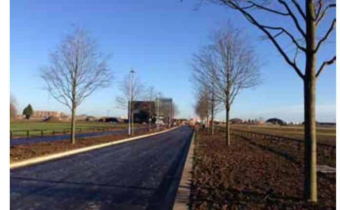
Boulevard between main entrance and Incubator building
