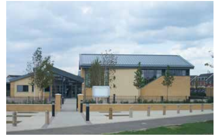
Primary School Precedent, Hampton, Peterborough - clear entrance and neat boundary treatment
