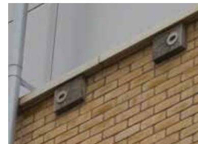
Swift boxes on buildings
