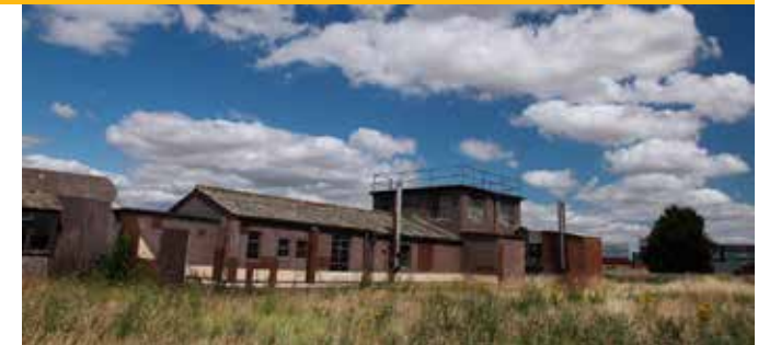
Listed Watch Tower Building
