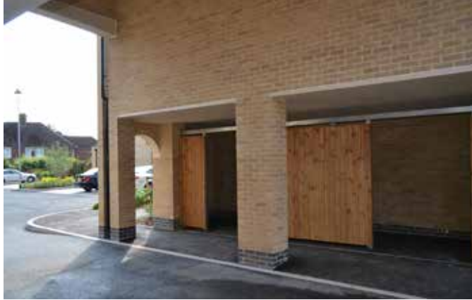
Precedent of bin storage, incorporated into residential design scheme at Primrose Lane, Huntingdon
