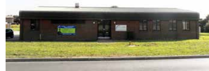
Figure 7d: Precedent example of reuse of existing buildings
