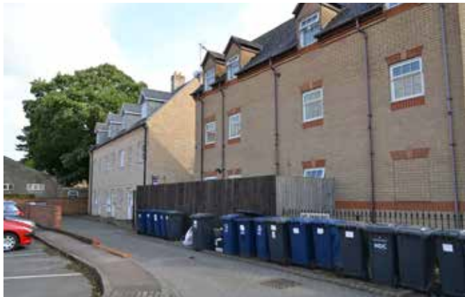
Precedent image of bins dominating the streetscene in a scheme that may have insufficient bin storage.
