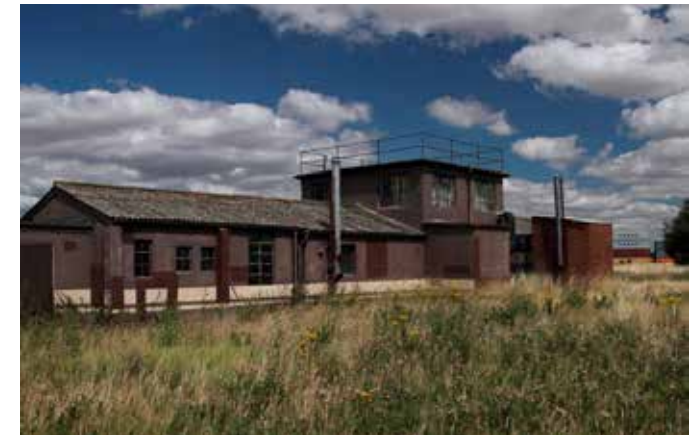
Listed Watch Tower – south west elevation
