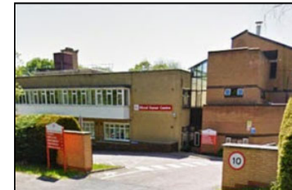
Blood Centre, Brentwood – Negotiated uplift from 22 to 55 units with planning, Disposal receipt secured £7.02m against c£2.5m investment
