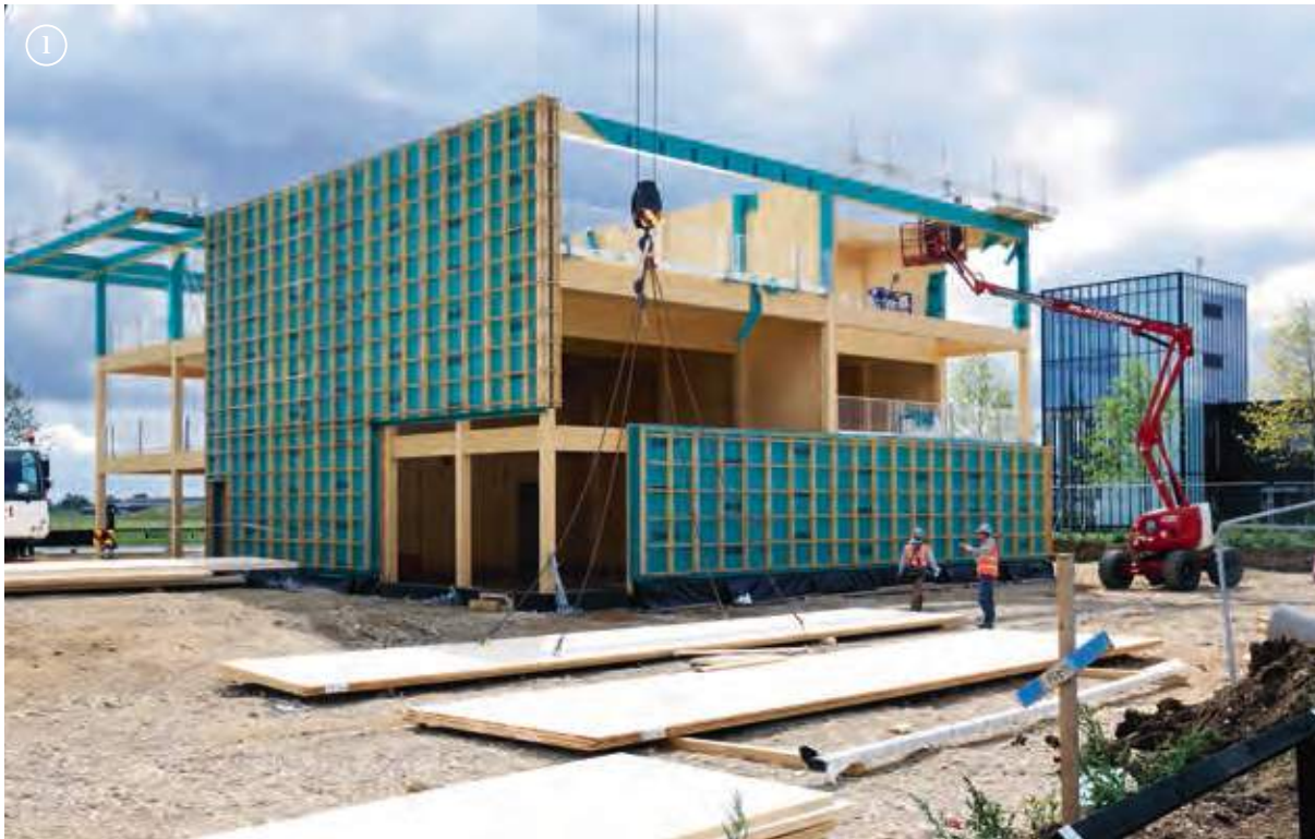
1 The Club building's timber frame 2 Electric bike scheme at Alconbury Weald
