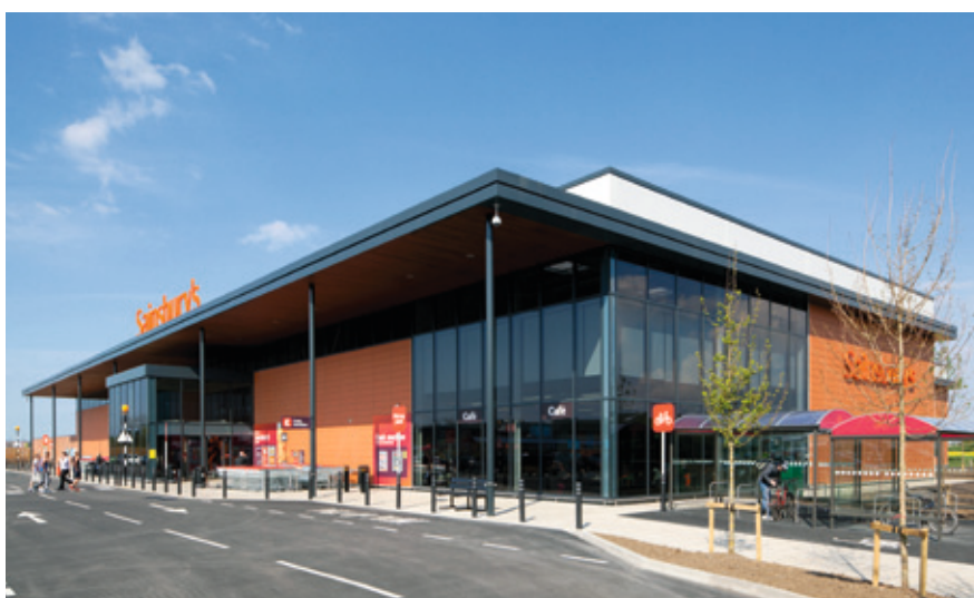
Completed Sainsbury's store at Sedgefield, County Durham.
