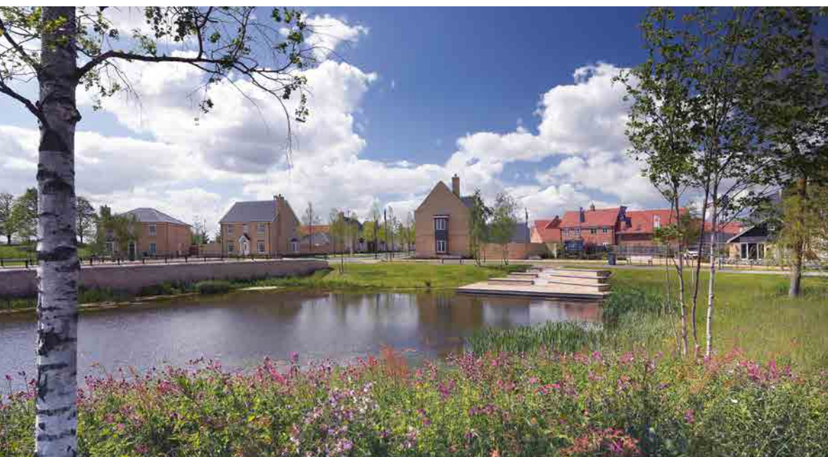
The causeway and lake at the entrance to Phase 1 of Alconbury Weald this summer.
