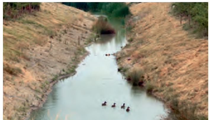
Sustainable urban drainage running through an ecology corridor at Rugby.
