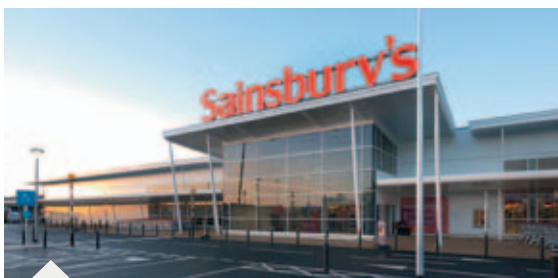
Built and fitted out in 30 weeks.
