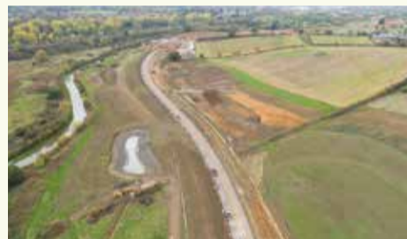
Link Road under construction
