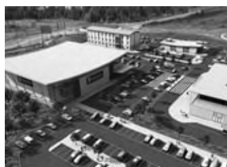
Middlesbrough Gateway, Middlehaven ↓
