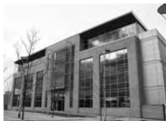
Gateshead, Baltimore House Baltic Business Quarter ↓
