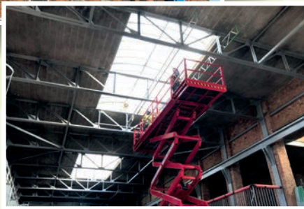
Work is underway to restore the Grade-II listed building
