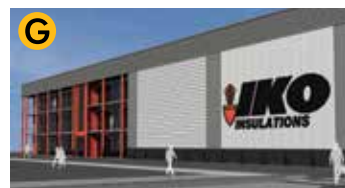
G IKO Insulation manufacturer. UK headquarters (Dec 2017)
